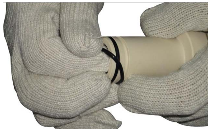
Figure 2.15 Adaptor seals installation
